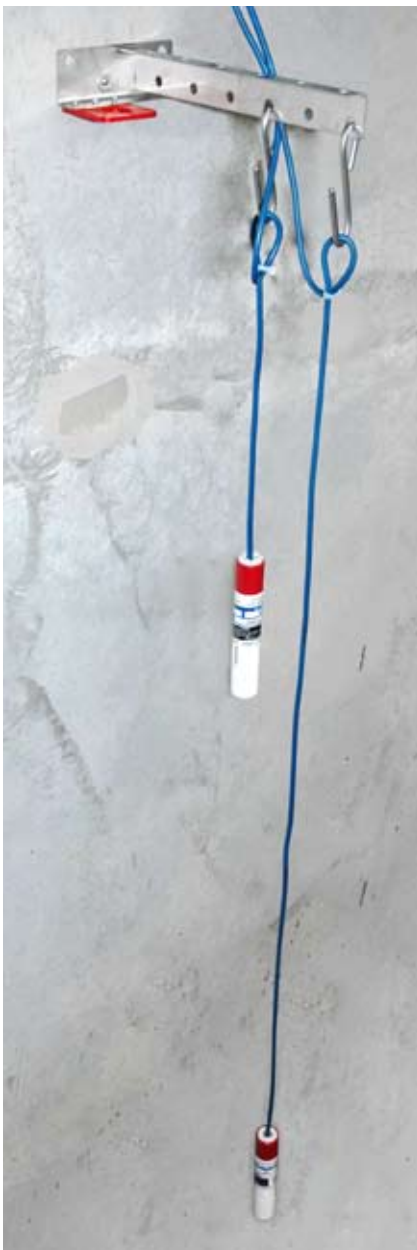
Two single sensor probes (e.g. from a sump pack), with optional extender bracket.
